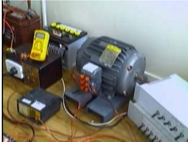
Panacea's 50 hertz 5 HP Baldor motor modified to run in RV mode to give .8- 1.13 HP for energy saving applications.
