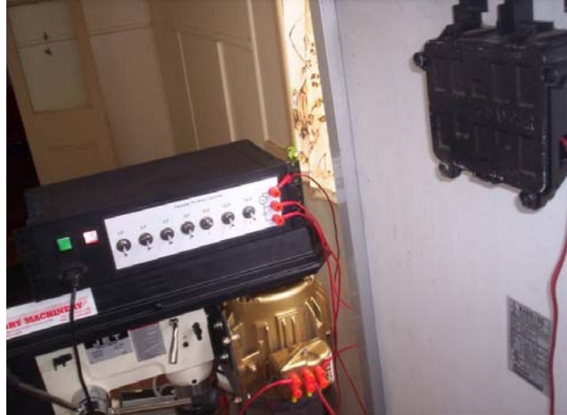
Panacea-BOCAF's 50 hertz RV Drill with 120 watt solar panel pictured right
